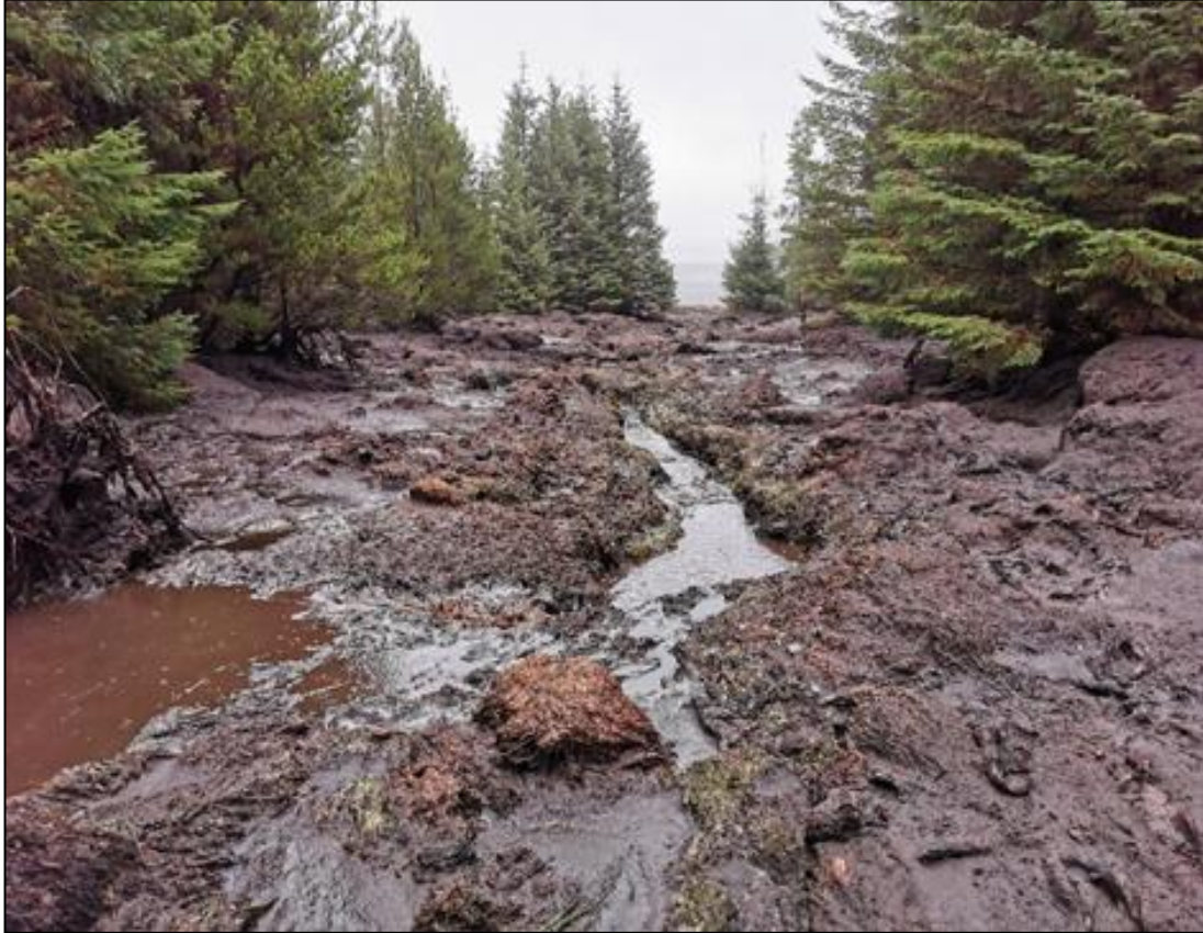
Plate 3-10 Shruhangarve immediately after the November 2020 Peat Slide
